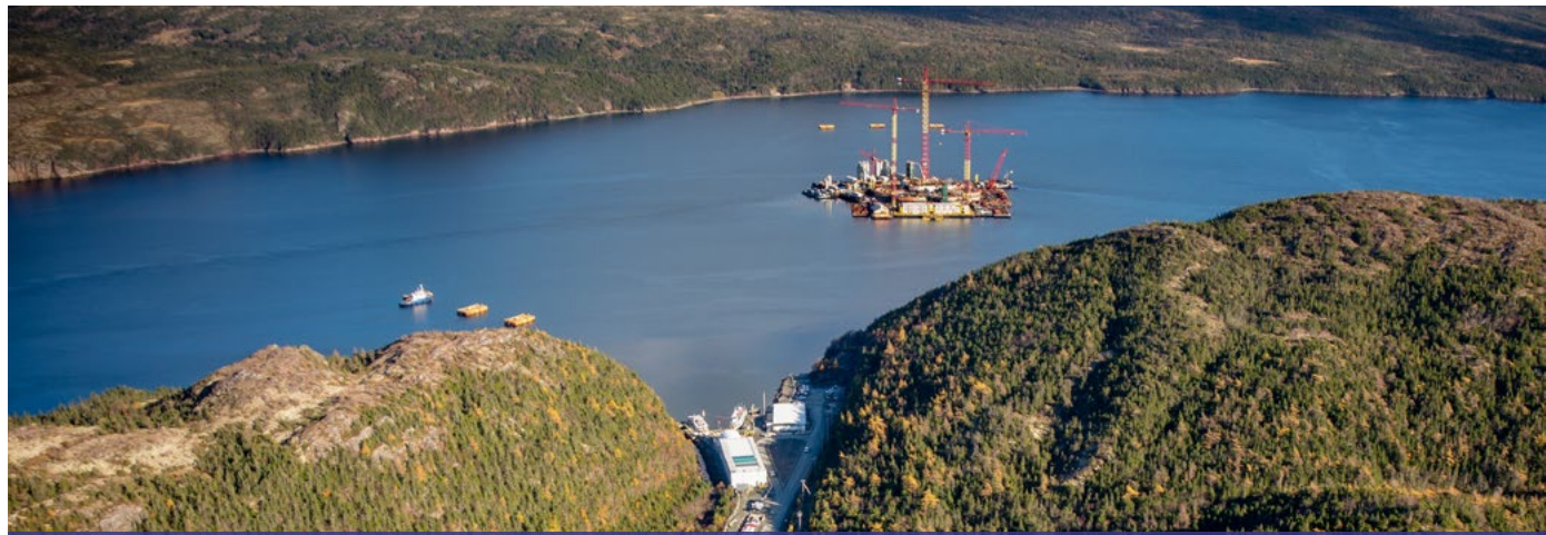
The Hebron project under construction in Newfoundland and Labrador, Canada.
