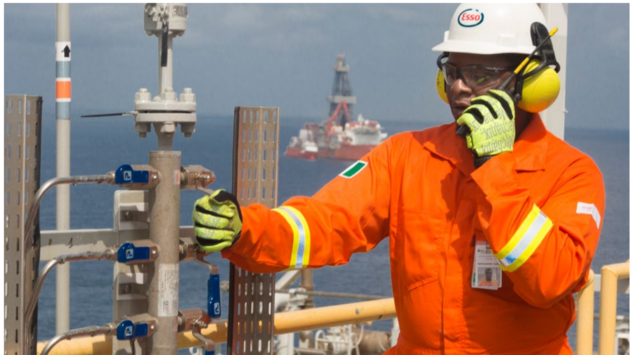
Kanu Okechukwu, a production operator for Esso Exploration and Production Nigeria Limited, opens a manual valve to supply compressed air to equipment at the Erha North phase two project in Nigeria.
