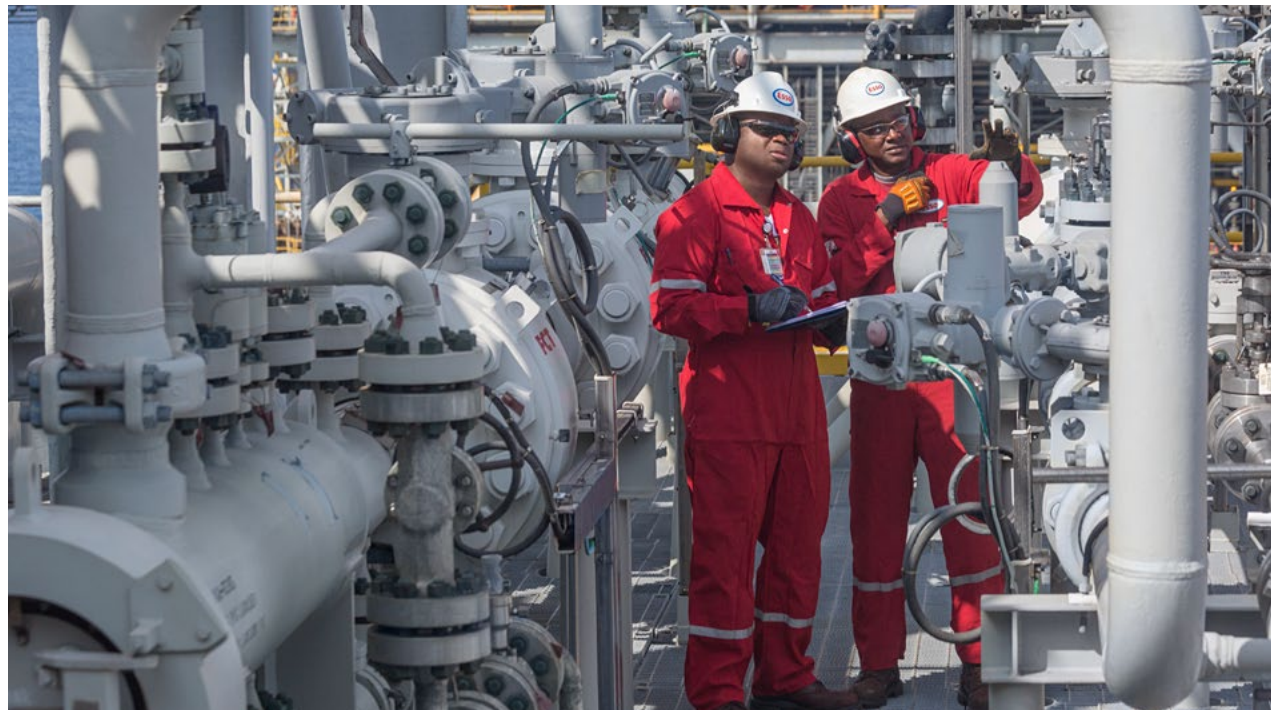
Local personnel Luis Almeida and Diwalter Fortunado inspect equipment at our Kizomba project in Angola.
